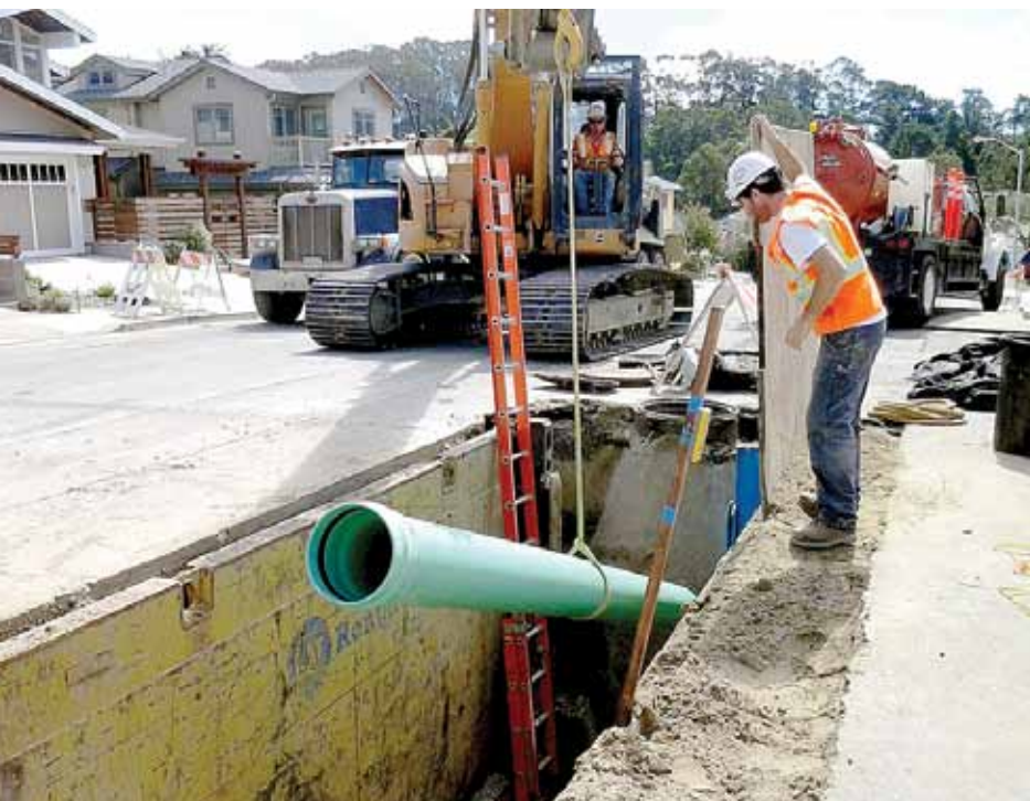
San Bruno Sewer Pipe Lines Phase III
