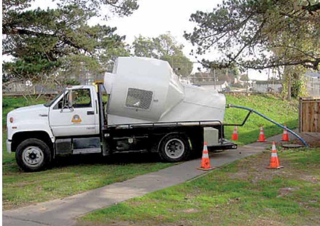
A Mechanical Rodder Truck Removing Roots in a Sewer Main
