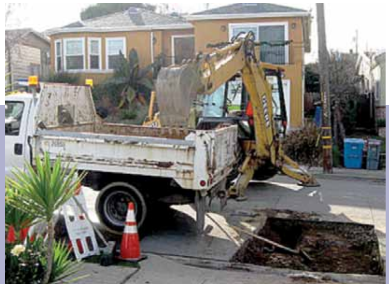
A sewer lateral pipe excavation
